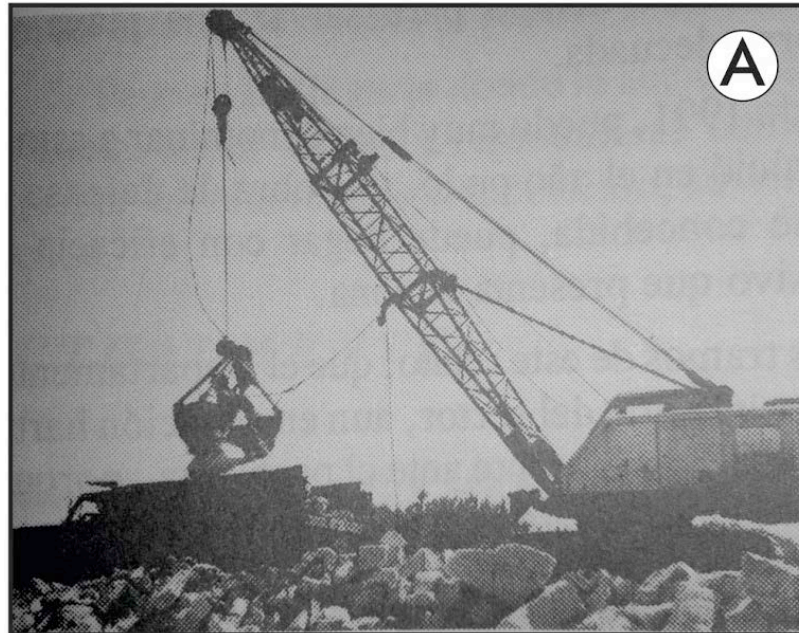
Figure SI-IVa - Constructions of the breakwater in 1991. Souce: Langrange, 1993
