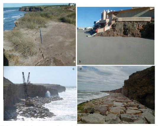
Figure 4 - Cliffs from Mar del Plata (38° S, see figure 1 for location). a) Fracture cracks on the top of the cliffs. b) Sea-side constructions are usually located attached to the cliffs composed of indurated siltstones. c) Rock revetments under construction. d) Armored structures are today protecting some cliffs.
