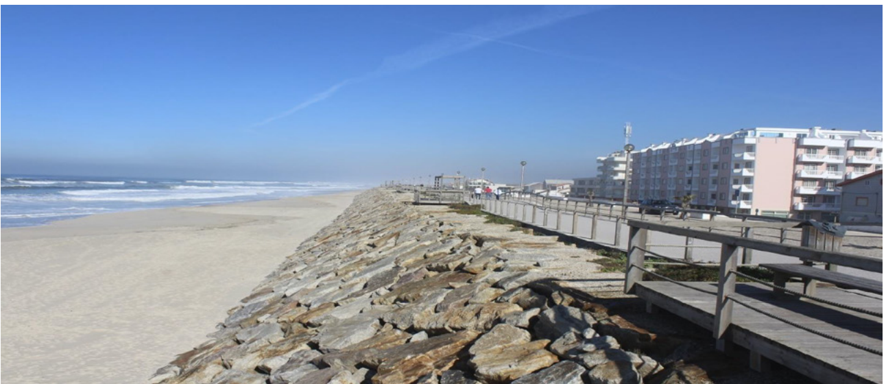
Figure 1. View of the longitudinal frontal defence structure of Vagueira beach (Rosa, 2021).
