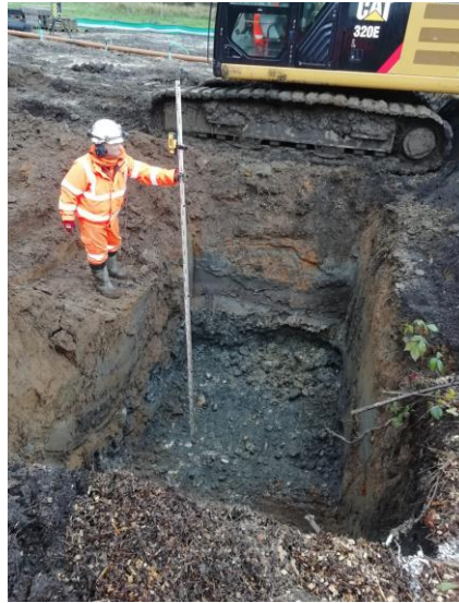
Fig.6 Trial Pit prior to Blockade
