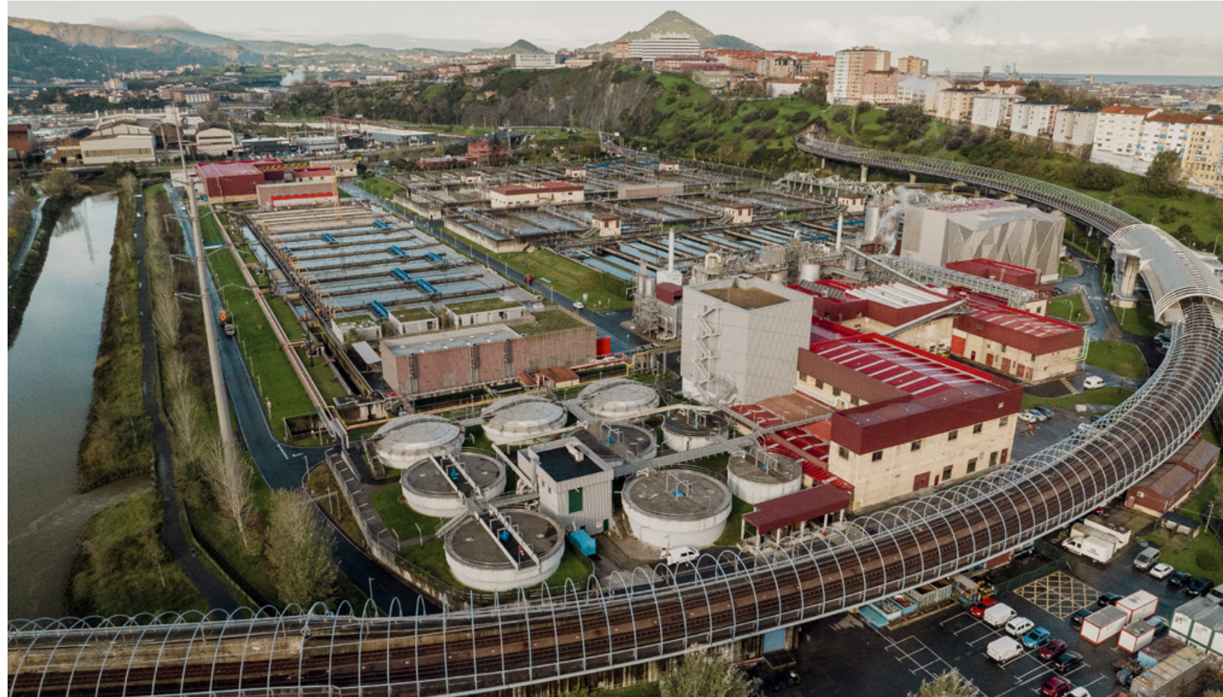
Galindo WWTP, in Sestao, Bizkaia. ©González-Cebrián
