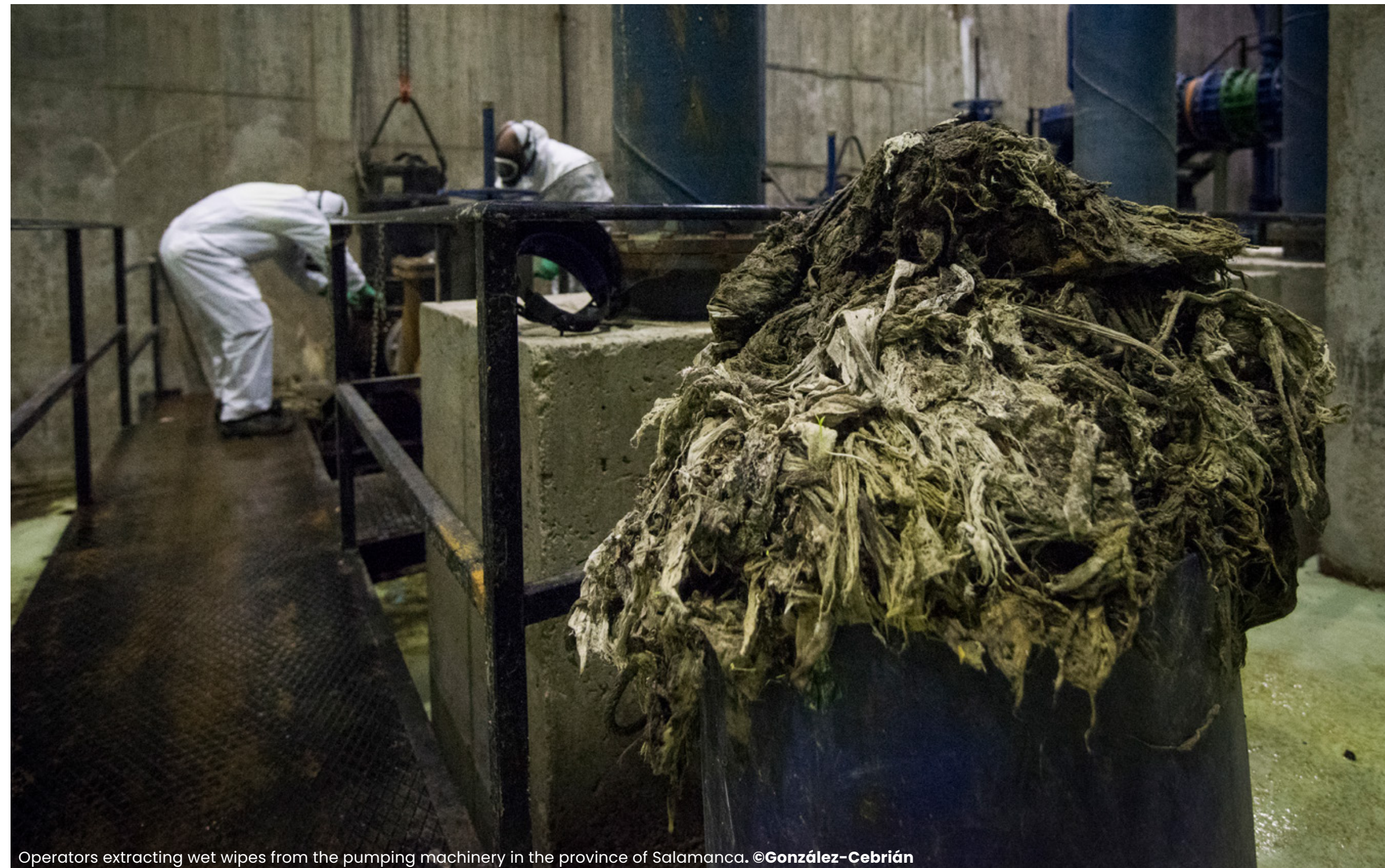
Operators extracting wet wipes from the pumping machinery in the province of Salamanca. ©González-Cebrián
