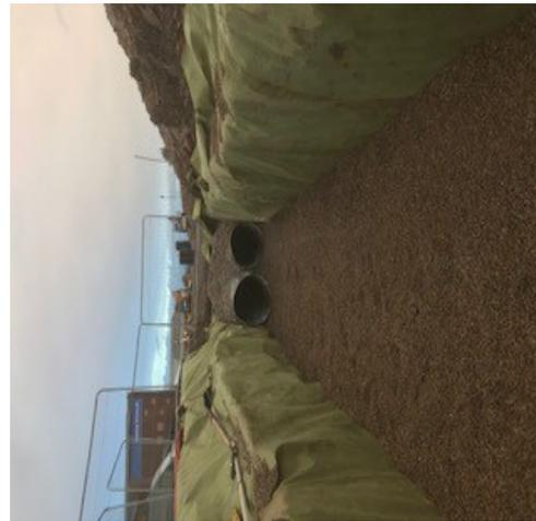
Fig. 2. Backfilling of attenuation pipes.
