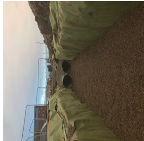
Fig. 2. Backfilling of attenuation pipes.
