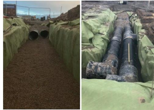
Figure 3. Perforated pipes within attenuation trenches.
