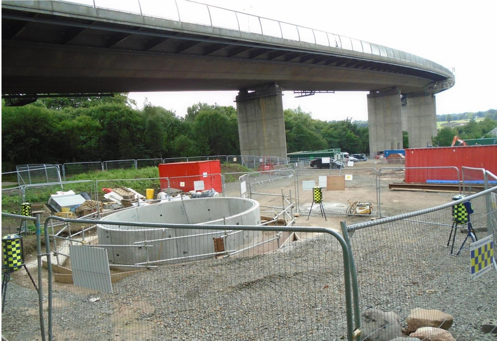
**Shaft construction requiring dewatering close to Erskine bridge piers**
