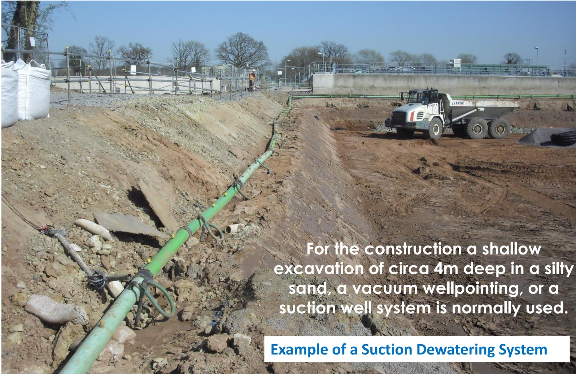
For the construction a shallow excavation of circa 4m deep in a silty sand, a vacuum wellpointing, or a suction well system is normally used.
