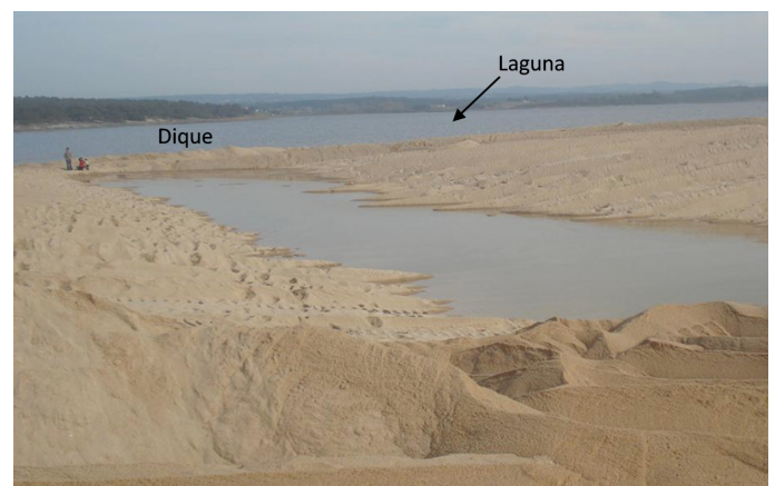
Figura 3. Dique (na margem interna da barreira) e vala escavada durante a operação de abertura artificial da embocadura. Figure 3. Sandy dike on the internal margin of the barrier, and excavated trench during the opening works of the artificial inlet.
